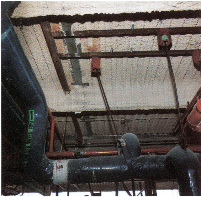
Figure 11. Pipe support rods were displaced which caused the piping to distort. The pipe distortion is expensive to repair (8th floor location, 8 stories, approximate maximum seismic excitation - 0.36 g horizontal, 0.22 g vertical).
