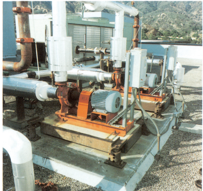
Figure 8. The seismic snubbers are built into the vibration isolators. The system was properly adjusted and withstood the effects of over 2 g input and remained operational. The mounting type is Mason SSLFH (roof location, 7 stories, approximate maximum seismic excitation - 2.3 g horizontal, vertical n/a).
